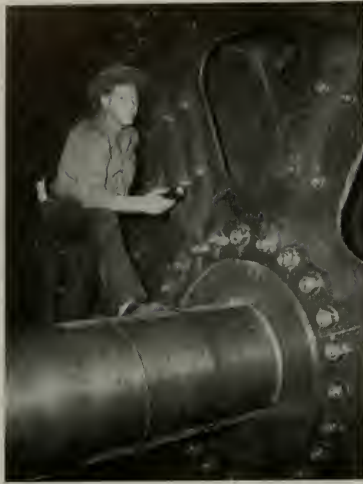
Ed Harris, manager of Uhlin Machine Works, Inc. This view shows upper half of reinforcing plate of main motor spider on the Fort Jupiter.
